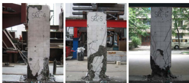
图1 型钢混凝土柱在水平往复荷载下的破坏形态 Fig.1 Failure patterns of SRC columns under horizontal cyclic loading
